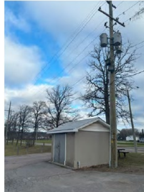
Photo B01: Block Building and 3 x Pole mounted XFMR Incoming Power Service
