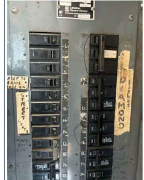
Photo B02: Existing Panelboard 'B' feeds Tye Field, Parking lot and street lighting
