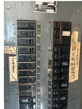
Photo T03: Block Building Panelboard 'B' 3 x 70A, 3P circuit breakers feeding Tye Field light standards
