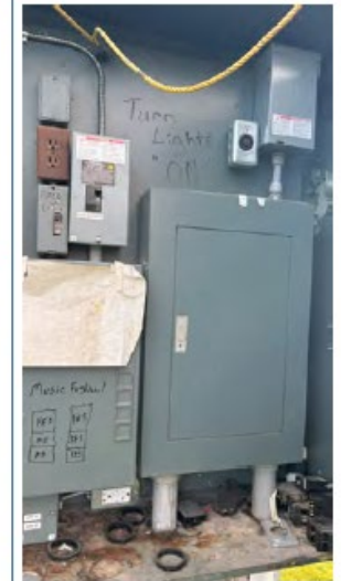
Photo R04: Rusheleau Field Enclosure Panelboard and Contactor
