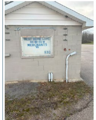
Photo T04: Block building, 3 x 2" conduits transition underground towards Tye Field
